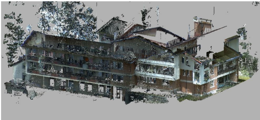
Fig. 9. Point cloud obtained by terrestrial laser scanning
