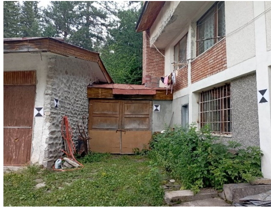
Fig. 5. Placed paper marks on the facades of the object
