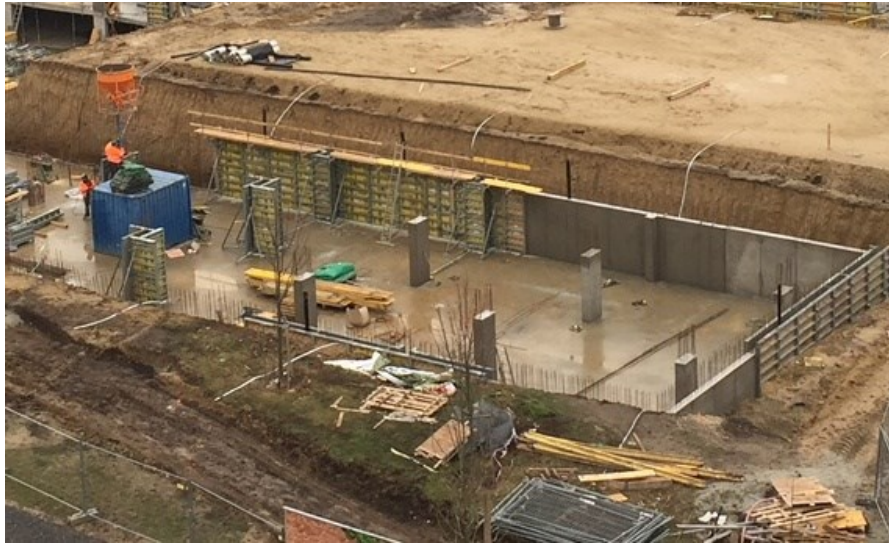
Fig. 2. Realization of walls and columns on the foundation plate.
