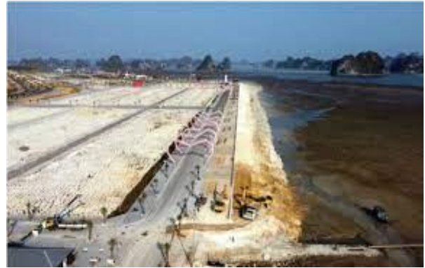
Fig. 2. Leveling activity for sea encroachment project at Phuong Dong urban area, Van Don - Quang Ninh [9].
