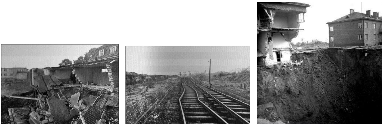
Fig. 2. (left) Garages in Karol Swierczewski Street were completely collapsed by a huge sinkhole on 5 th August 1977, (middle) railway tracks were broken in the Wapno village [25], (right) A huge hole in the Wapno village, which was allegedly caused by land subsidence triggered by mining exploration in the Tadeusz Kościuszko salt mine [26].
