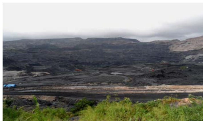
Phot. 1 General view of opencast coal mine Coc Sau [7]
