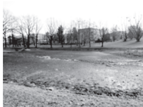
Fig. 3 A dry reservoir intended for area fire protection
