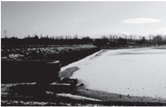
Fig. 2 A water supply reservoir designed for the supply of industrial water
