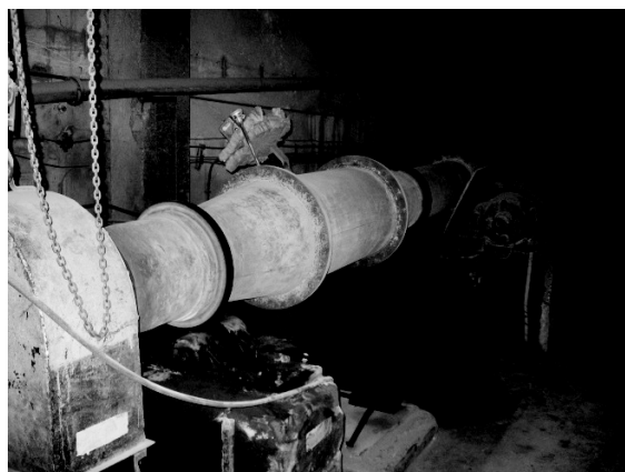
Fig. 3. Rotary furnace for sintering of light aggregates
