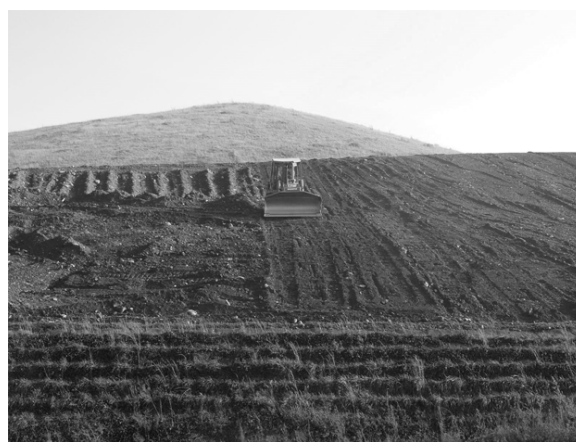
Fig. 10. An example of revegetation of the Central Heap of JŠM [3]
