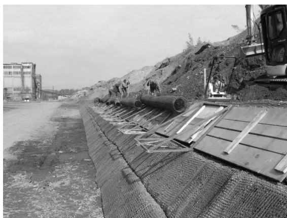
Fig. 2. The geogrid-reinforced structure [3] Rys. 2. Struktura wzmocnionej geokraty [3]
