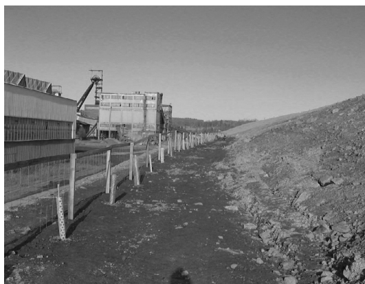
Fig. 7. The geogrid-reinforced structure with a retaining grid and shrub planting [3]
