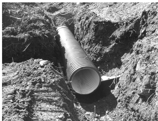
Fig. 9. Plastic corrugated pipes [3]
