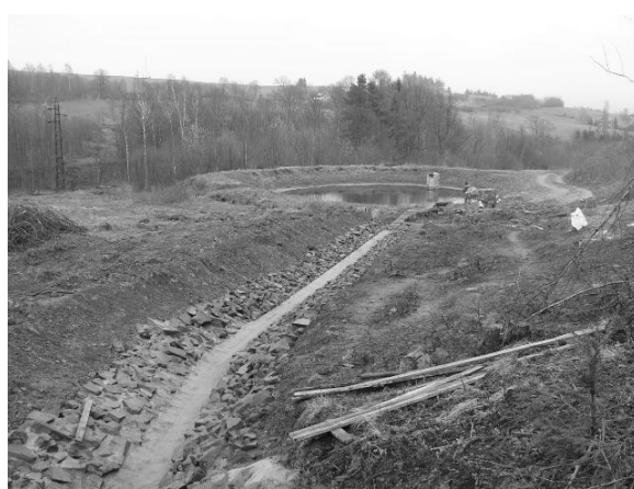
Fig. 8. Ditches are reinforced with stones [3]
