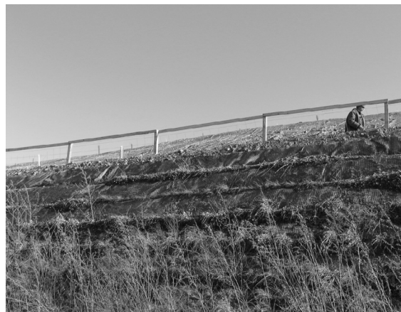
Fig. 6. The geogrid-reinforced structure with a retaining grid and shrub planting [3]
