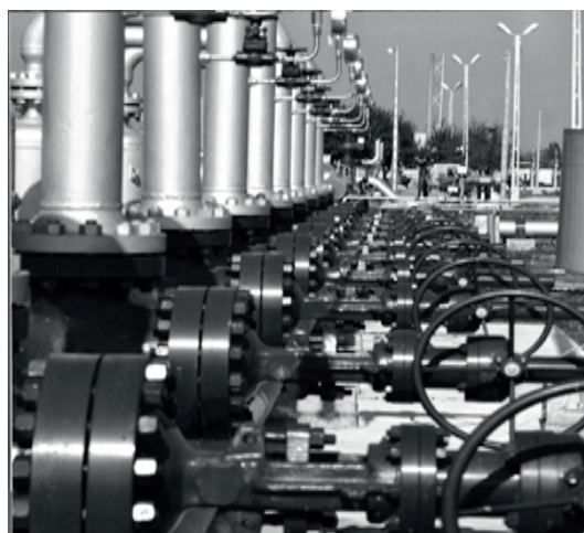
Fig. 1 The gas compression station
