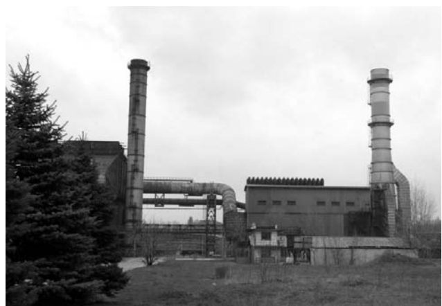
Fig. 2. View on the plant after implementation of resource-conserving technologies
